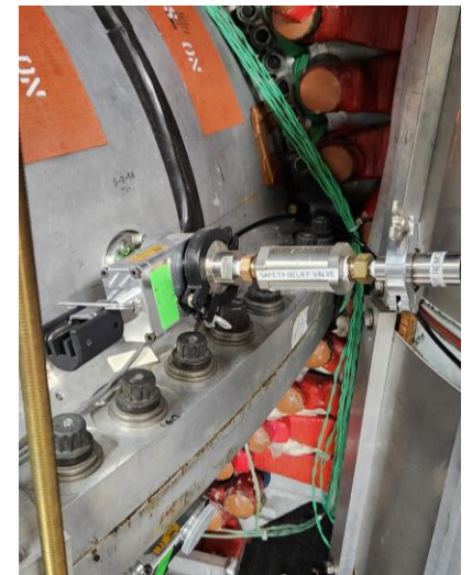
Safety overpressure valve
